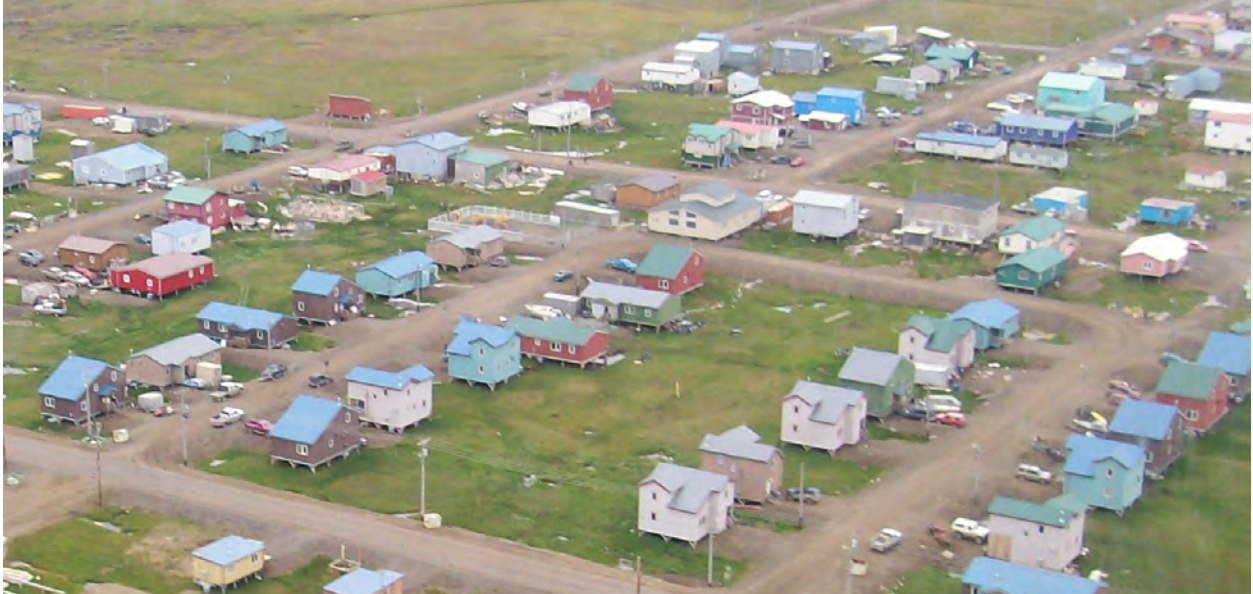
Image 17: All construction is on posts to protect permafrost from residential heating. Drift snow and high winds take a toll on paint and siding.
